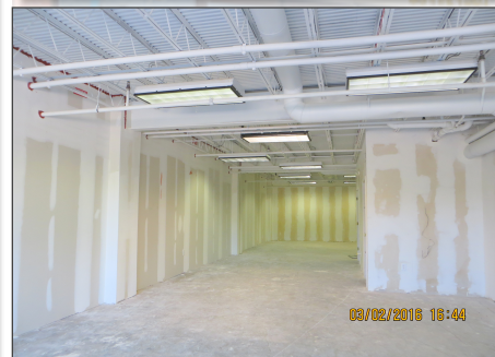
Renovations in Progress
